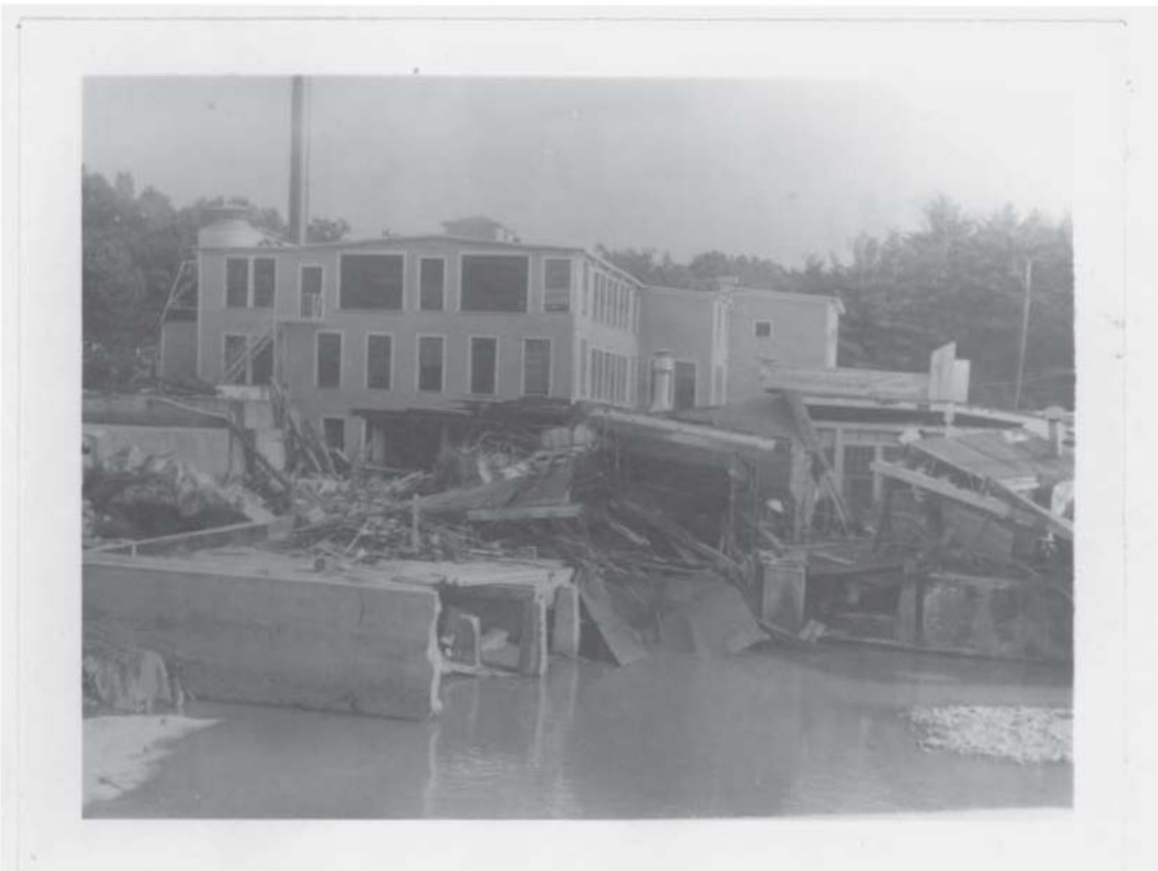
Fig. 3 Flooding During the 1955 Hurricane
