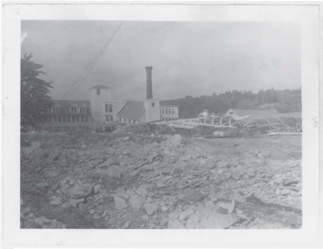
Fig. 2 Flooding During the 1955 Hurricane
