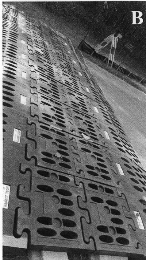
Figure 2. Hose-bridge from Turtle Plastics Inc. tested as a road-crossing structure for Storeria dekayi along Ridge Lake Road in Fox Ridge State Park (Coles Co., Illinois). (A) During construction, illustrating size relative to road and vehicles. (B) Hose-bridge construction and drift fencing complete.
