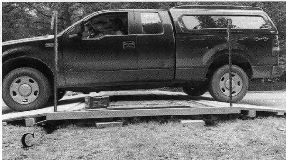
Figure 7. Images of modifications to the hose-bridge in 2015 on Ridge Lake Road in Fox Ridge State Park (Coles Co., Illinois). (A) Detail of cross section of ramp constructed to improve vehicle mobility while crossing. (B) Overall ramp construction view as approaching vehicle. (C) Vehicle traversing the hose-bridge structure with ample clearance provided by ramps.
