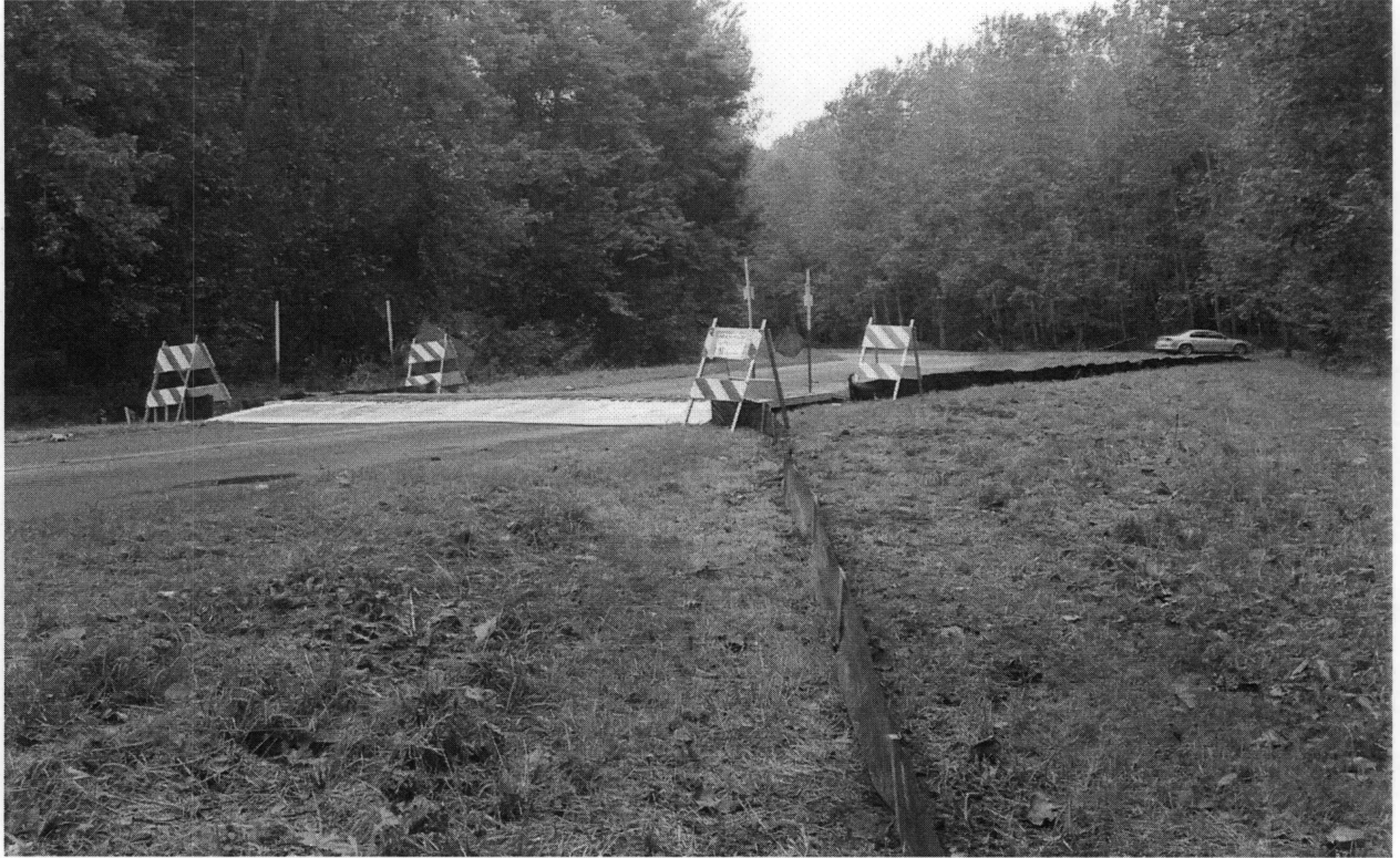
Figure 4. Drift fences built at both hose-bridge and control sites to direct flow of Dekay's Brownsnakes migrating across Ridge Lake Road to hose-bridge and control sites, respectively. Located in Fox Ridge State Park (Coles Co., Illinois)
