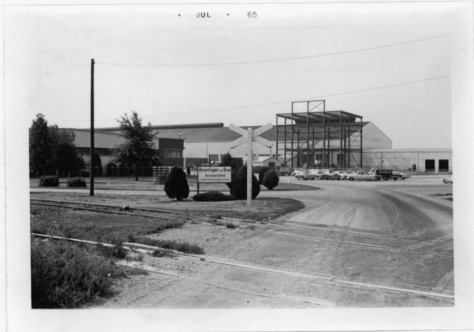
Fig. 2-17.--The north entrance of the Revere plant in Clinton.
