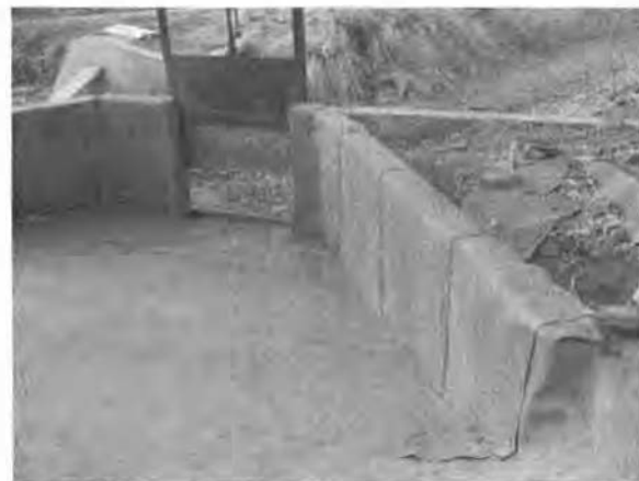
Figure 2- Repaired sides and bottom of basin [2]
