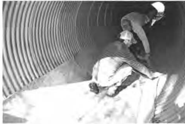
Figure 3- Installing the GCCM panels [3]
