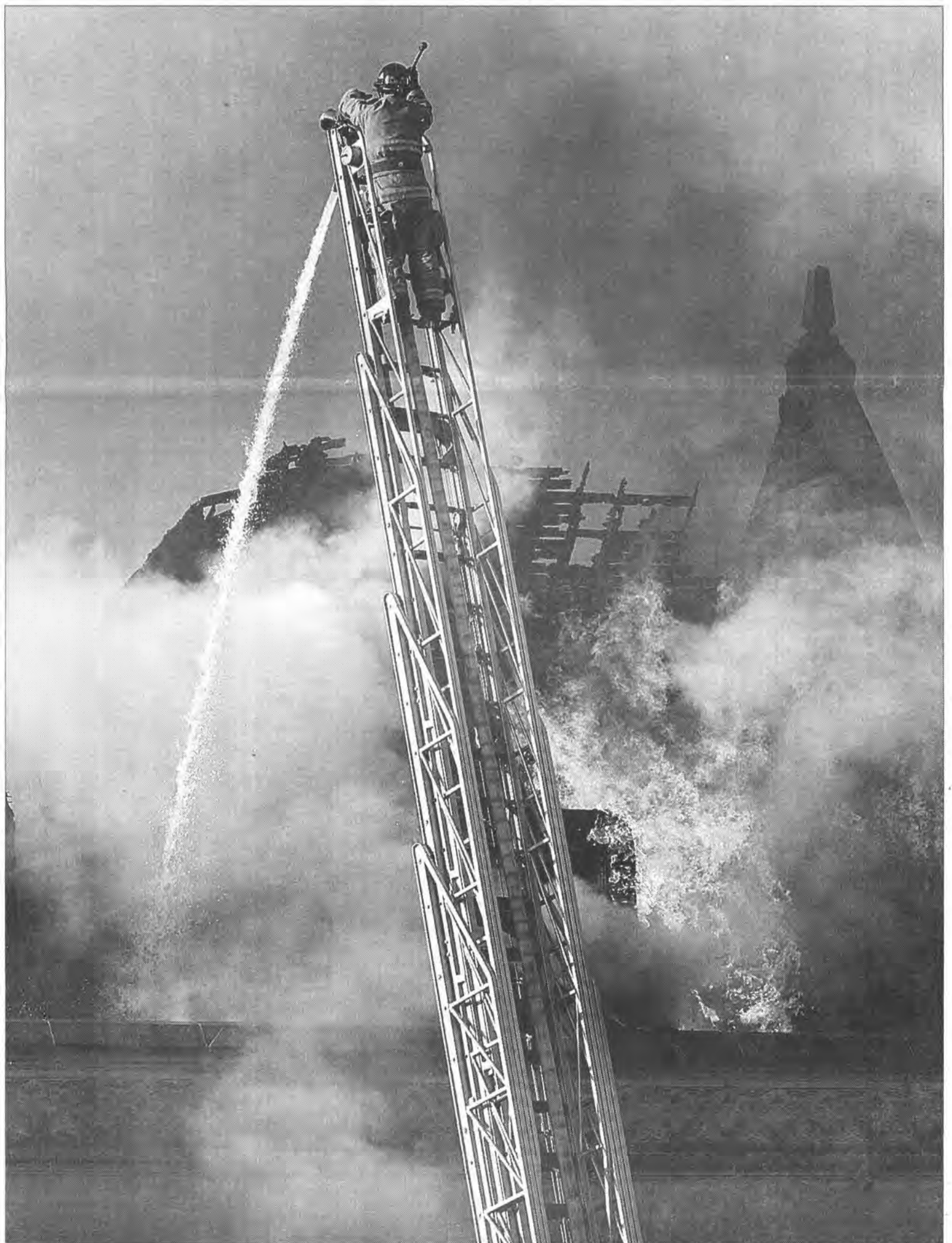
Charleston firefighter sprays water from an aerial truck on the southside of Blair Hall.
