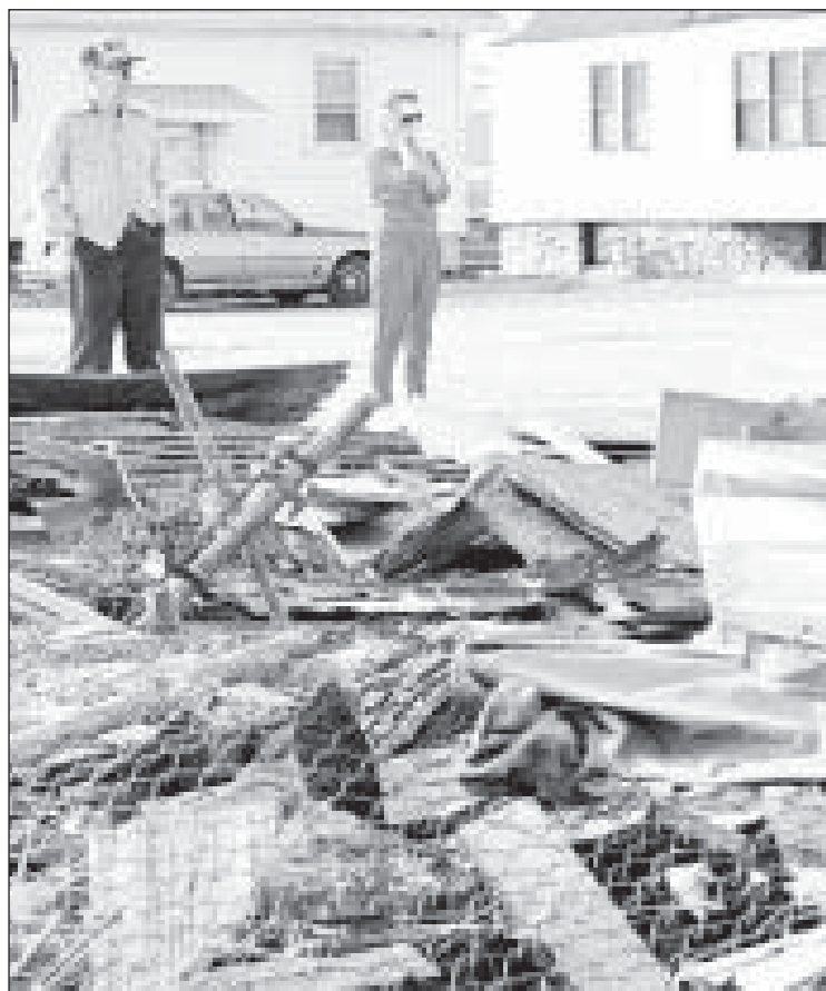
(Top) A truck on the 800 block of 17th Street and Walnut Street is buried under the fallen debris of Saturday's tornado. Residents of Mattoon are slowly cleaning up the area. Most of those affected by the tornado intend to stay in the area
