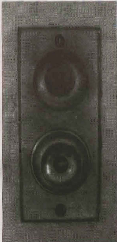
A speaking tube runs from the first floor to the second floor.
