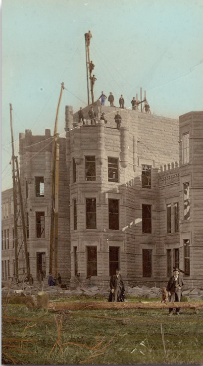
Old Main Under Construction, 1898
