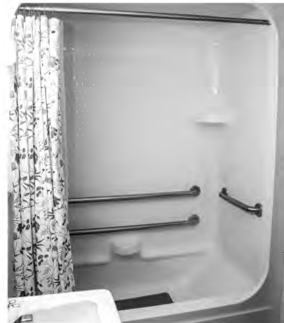
TOP RIGHT: Even getting in and out of the shower is difficult for Richardson, who lives in one-of-two accessible University Court apartments, because there is no outside handle to hoist themselves in and out. Richardson ends up using the side of the wall; they said the height difference is even hard for able-bodied people to get into the shower
