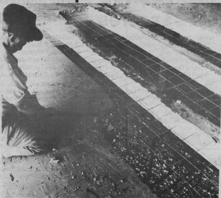
Workmen chop out floor tiles in the University Union Old Ballroom in preparation for pouring new concrete. A say was discovered in the floor last spring and raised questions about safety. (News file photo)
